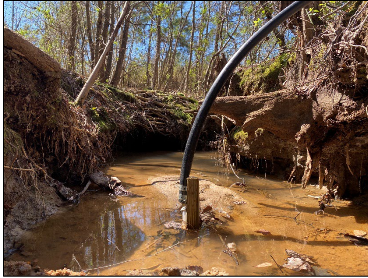
Figure 25. Evidence of unstable undercuts at MP467
